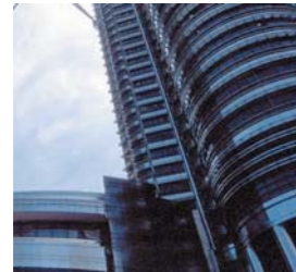
Cashier and car park systems
