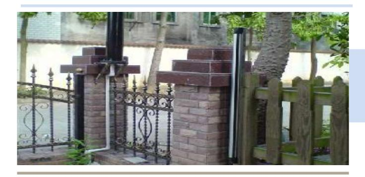
1, If there is intruder tried to climbe the fence into the house, it will buzzer and send signal to alarm control panel.
