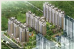
LARGE RESIDENTIAL COMPOUND
